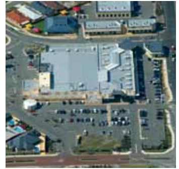
4. Southern River Shopping Centre, WA July 2011 - $25.5million
